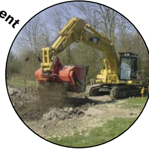
ALLU Screener Crusher - mixing/screening of soil and binding agent
