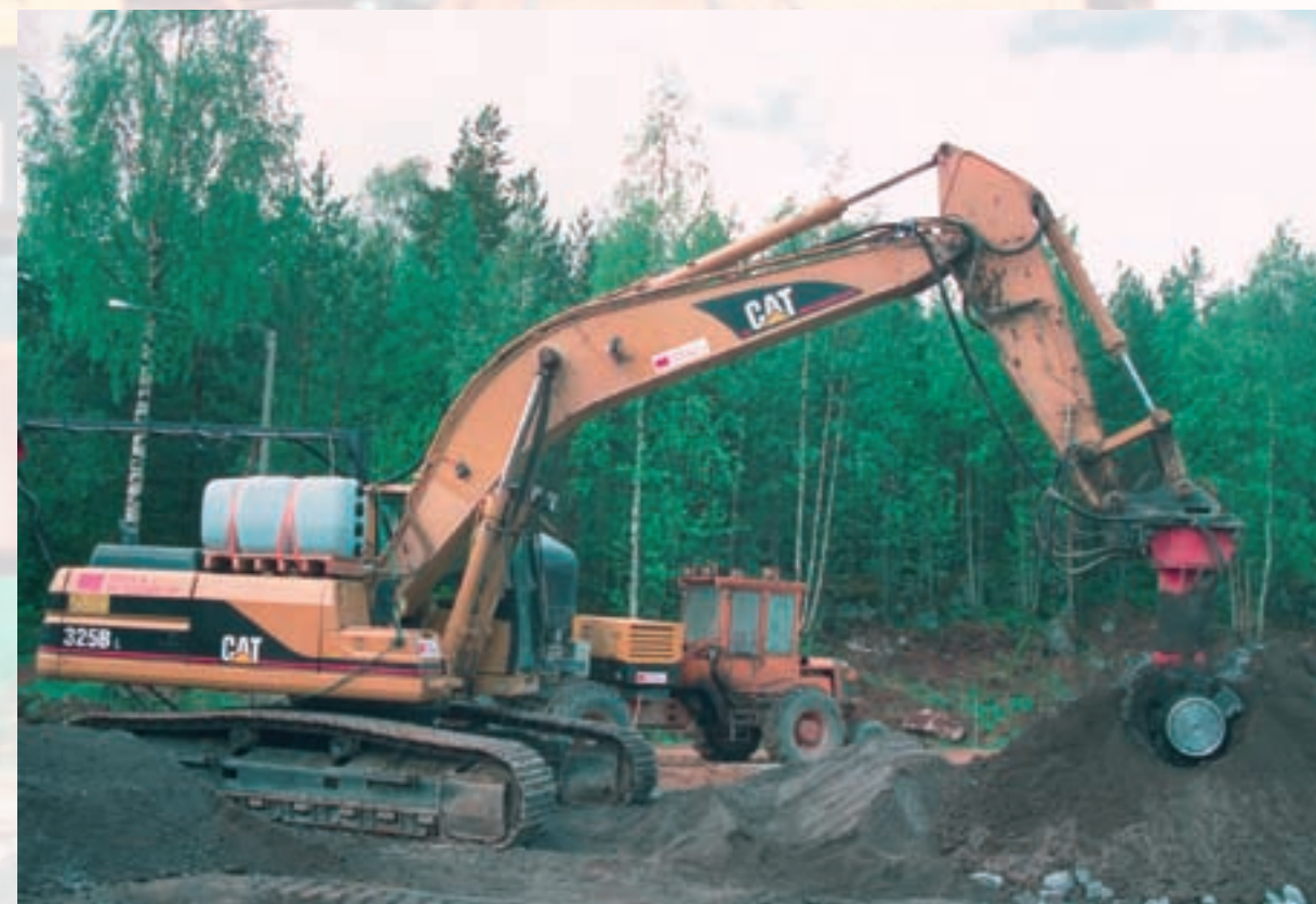
Ground improvement of the sport field in Luopioinen, Finland.
