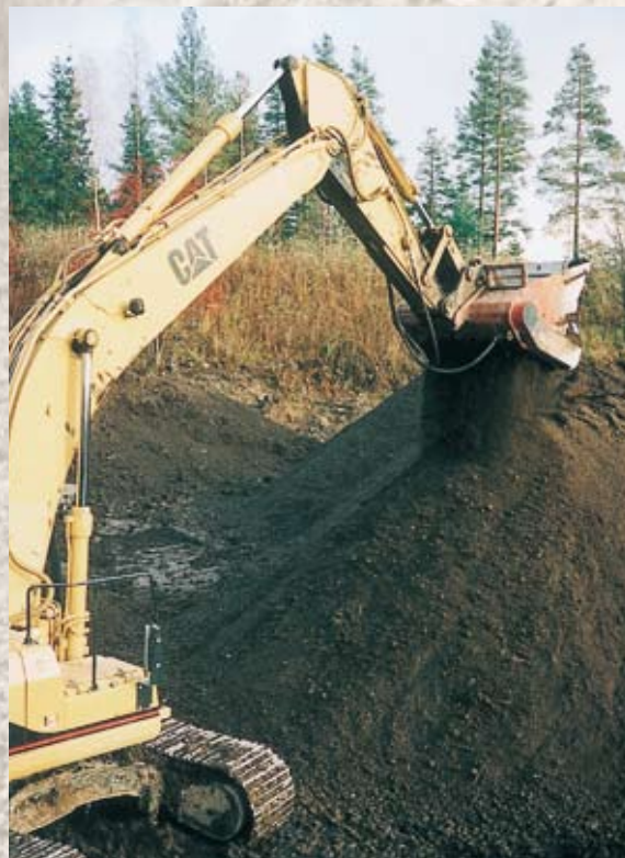
10. Stabilization of clay and contaminated soil.
