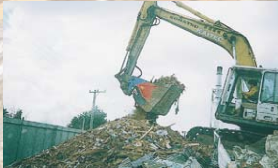
5. Construction waste and contaminated soil can be screened and crushed.
