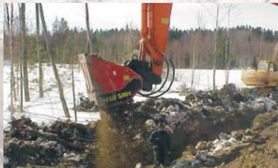
6. Screening and backfilling of pipeline trenches in one step operation.
