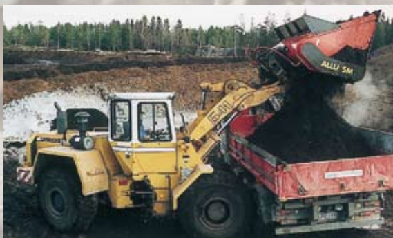
4. Screening and loading directly onto the truck in one step.
