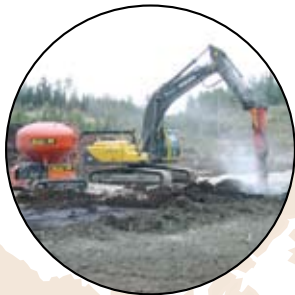
ALLU Stabilisation System - to strengthen and solidify different kind of soft materials
