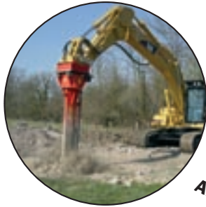
ALLU PM Power Mix - mixing soil and binding agent in mass stabilization
