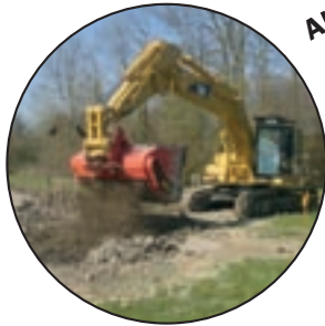
e.p.m - Powder Spreader - spraying of binding agent
